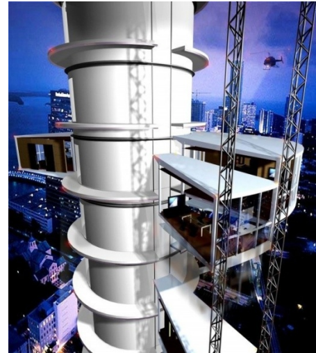
Fig. 2: Modules are assembled around the central core of the tower. Source: Infinity studio, 2007
